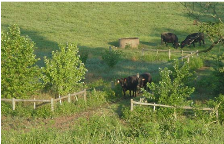
A culvert stream crossing, watering trough and stream fencing in Damascus, MD with CREP streamside forest buffer.
